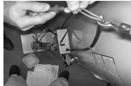
Checking continuity of upper sensor wire harness.
