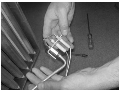
Step 17: Pilot removal for servicing.
