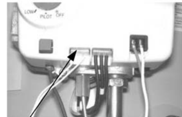
Chamber Door Temperature Sensor Wire Harness
