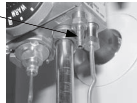
Pressure Tap Shown Installed
