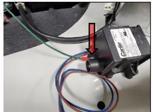
Step 8: Place ground wire loop terminal over mounting flange. Spark rod must be properly grounded to operate correctly.
