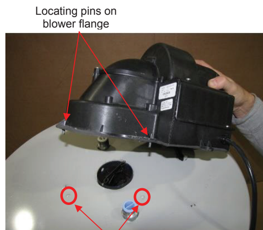
Pin location holes in jacket head
