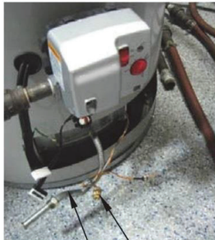
MAIN BURNER FLEXIBLE FEEDLINE PILOT FEEDLINE
