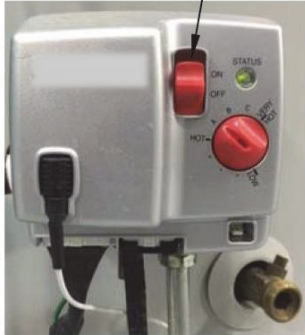
GAS CONTROL SHOWN IN THE "OFF" POSITION
