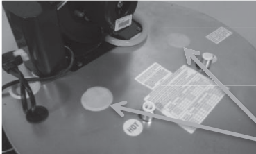
Anodes are located under caps
