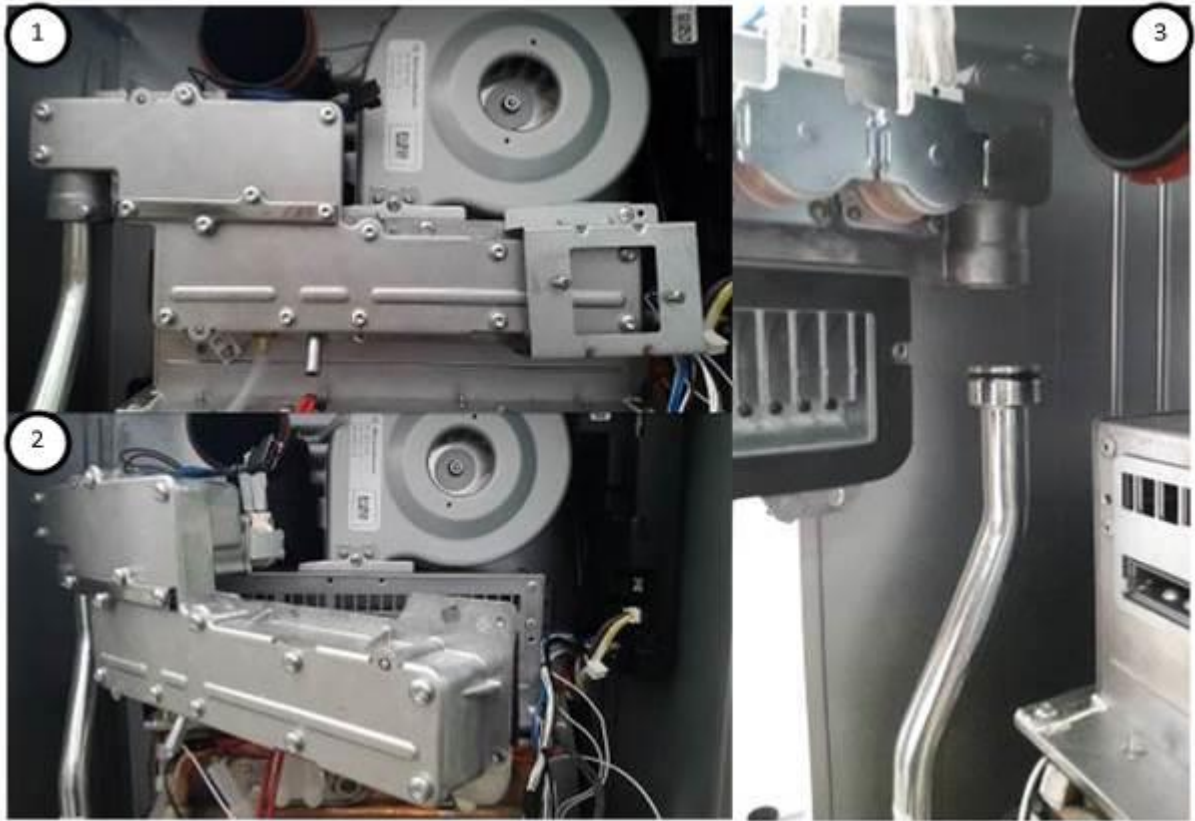
Figure 15 – Disassembling the manifold from the heat cell
