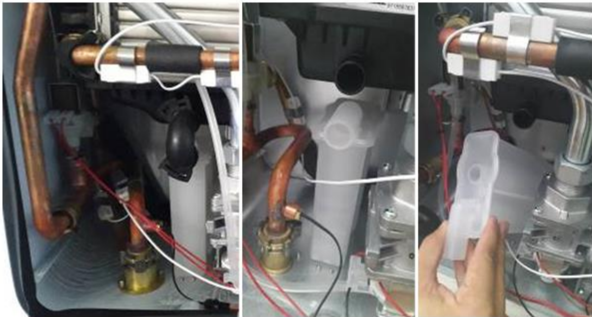
Figure 13 – Disassembling the Condensate Siphon from the Unit
