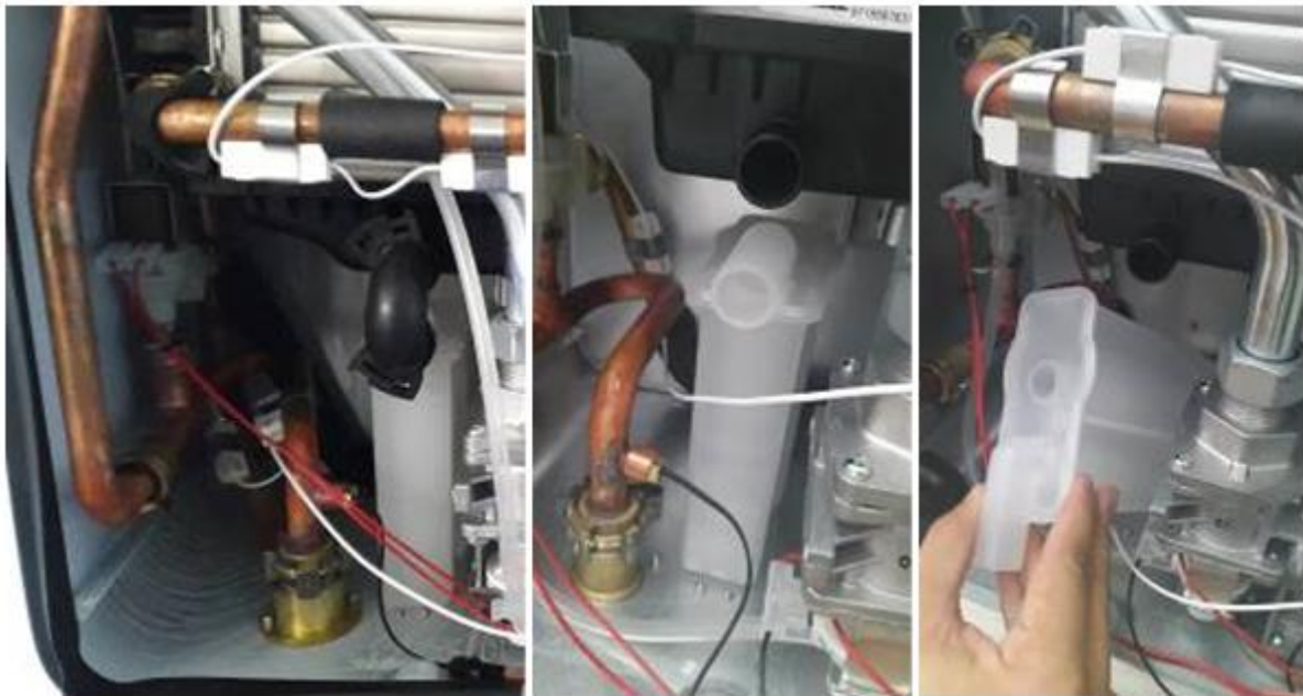
Figure 13 – Disassembling the Condensate Siphon from the Unit
