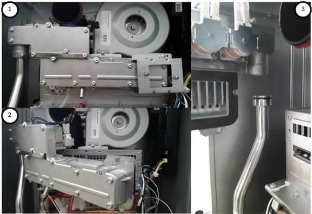
Figure 15 – Disassembling the manifold from the heat cell
