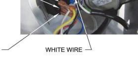
Step 11. Remove the White wire in the damper housing from its location. Connect the ¼" White female connector with the piggy back connector on the relay harness in its place.
