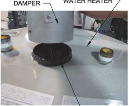
WATER HEATER TANK FLUE
