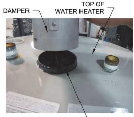
WATER HEATER TANK FLUE
