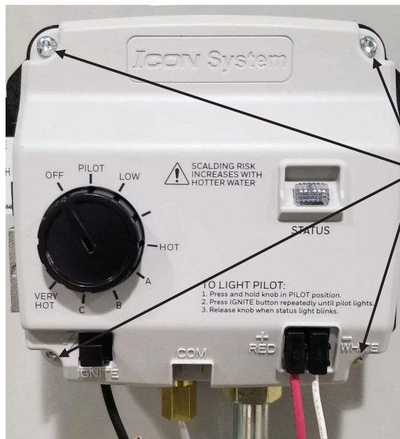
Gas control screws
