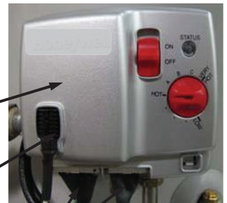
Spark igniter/flame sensor wire
