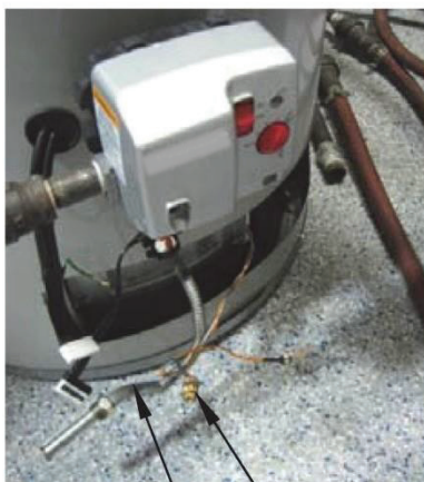
MAIN BURNER FLEXIBLE FEEDLINE PILOT FEEDLINE
