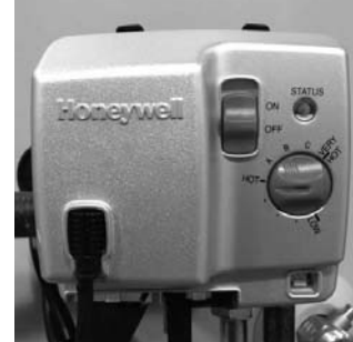
Gas Control shown in the “OFF” position
