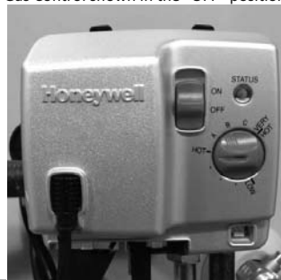
Gas Control shown in the "OFF" position
