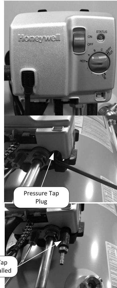
Gas Control shown in the "OFF" position
