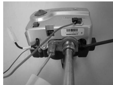
Gas Control shown in the "OFF" position
