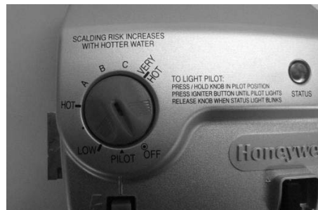
Gas Control shown in the “OFF” position
