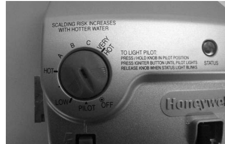
Gas Control shown in the “OFF” position
