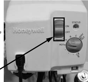
Gas control power switch
