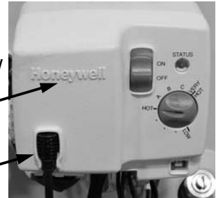
Spark igniter/flame sensor wire
