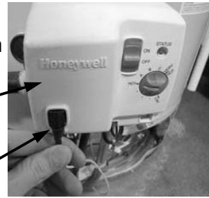
Spark igniter/flame sensor wire
