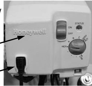
Spark igniter/flame sensor wire
