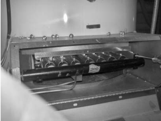
Step 7: Remove manifold bracket screws
