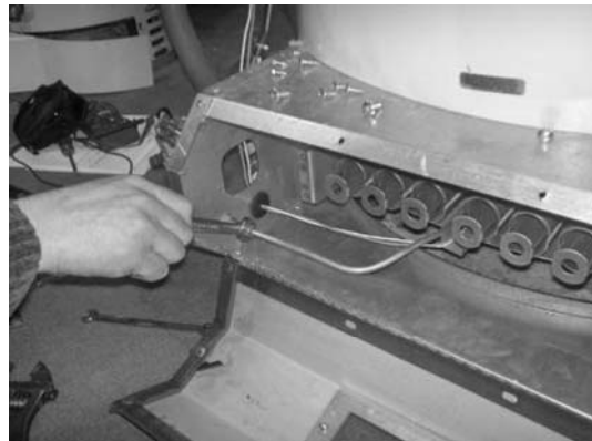
Step 10: Disconnect Pilot Tube Fitting from inside Burner Box
