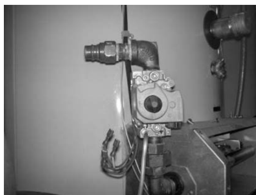
Step 4: Disconnect gas valve wires and pilot tube
