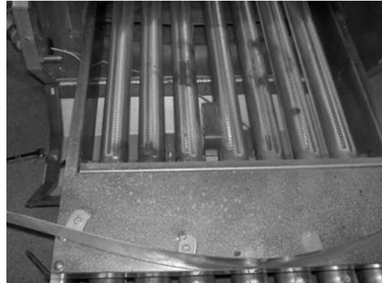
Step 14: Slide out burner assembly
