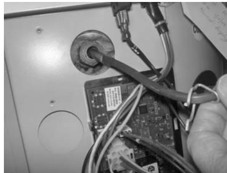
Removing lower sensor from well. Held in place by a clip fastened to well shoulder.
