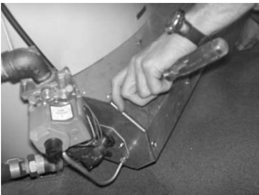
Step 1: Remove burner box cover screws
