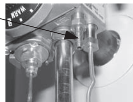
Pressure Tap Shown Installed
