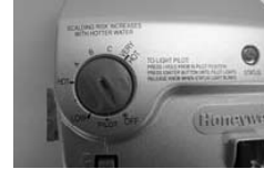
Gas Control shown in the "OFF" position
