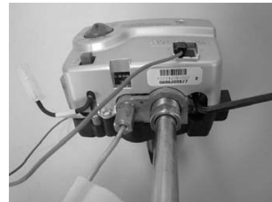
Gas Control shown in the "OFF" position
