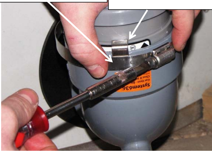
Flue Clamp Brackets on PVC Adapter Shoulder
