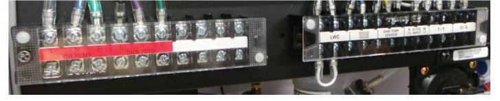
DHW and CH pump terminals for external pump are live 120V limited to 2.0 A. They operate respective to an external call (e.g T-T) for heat.
