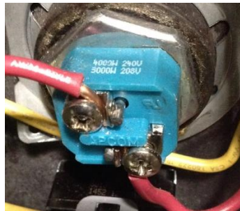
Figure 13. Example of Wattage/Voltage Marking on Element
