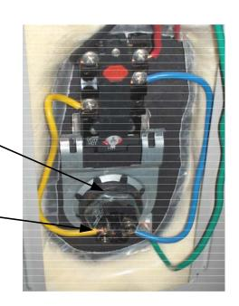
7. Remove element(s) from tank using 1½" deep well socket or wrench. Unscrew element(s) counter-clockwise to remove from tank.
