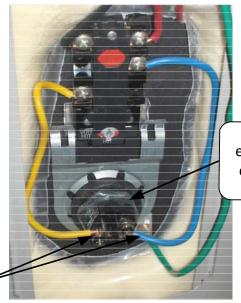
Thread element(s) clockwise into tank
