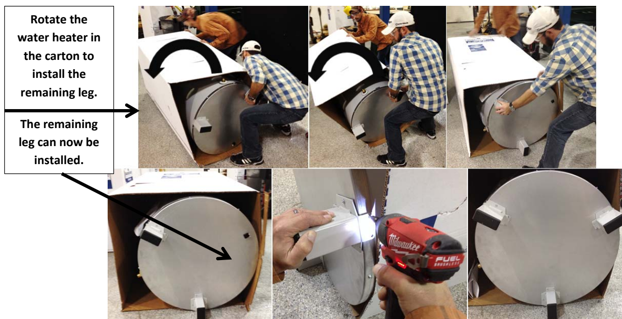
Figure 7: Accessing and installing the third leg.
