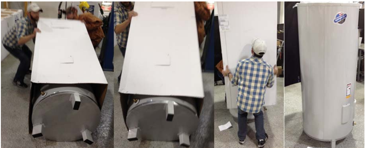
Figure 9: Lift the water heater into the upright position with two or more people.
